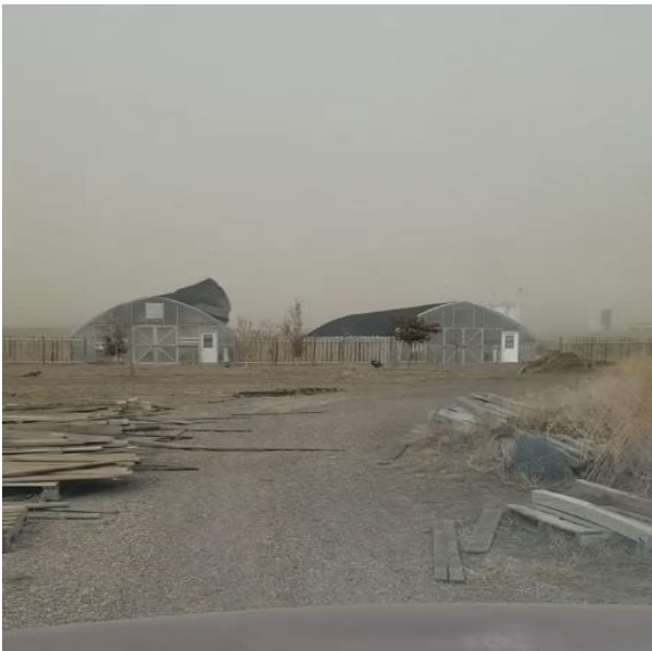
December dust storm & damage—Garden City—page 4
